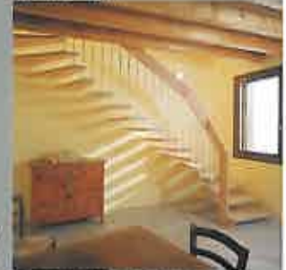
Open tread staircases
